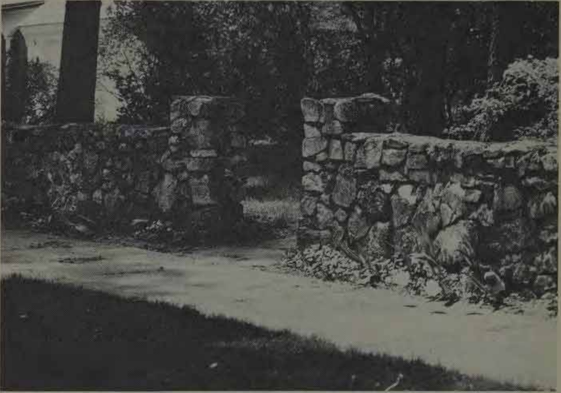
Chunky and irregular stones become a handsome mortared wall screen for a secluded city home.
