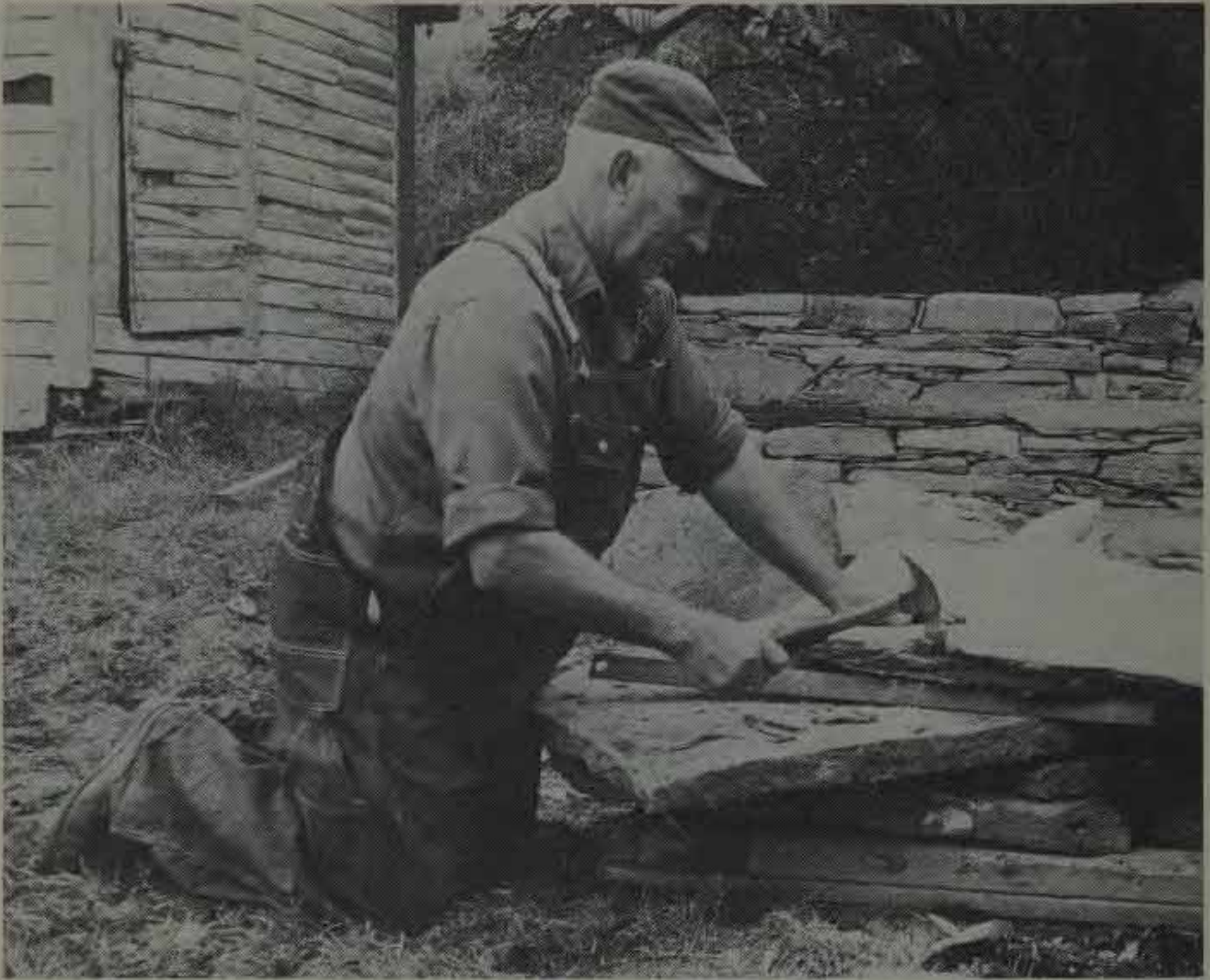
A ragged stone end is chipped straight atop an angle iron. The stone boat makes an improvised work bench.
