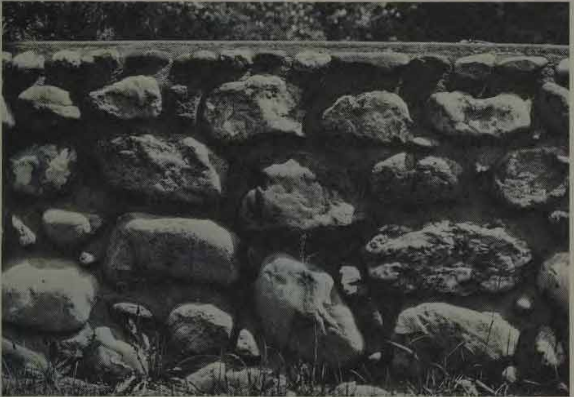
Wall built with big cobble stones cemented together.
