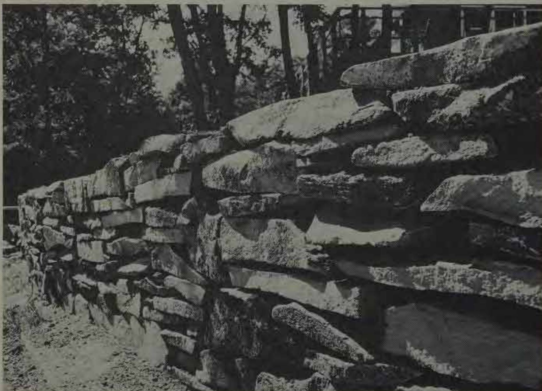
A completed wall. Note the use of the "one-over-two, two-over-one" principle.
