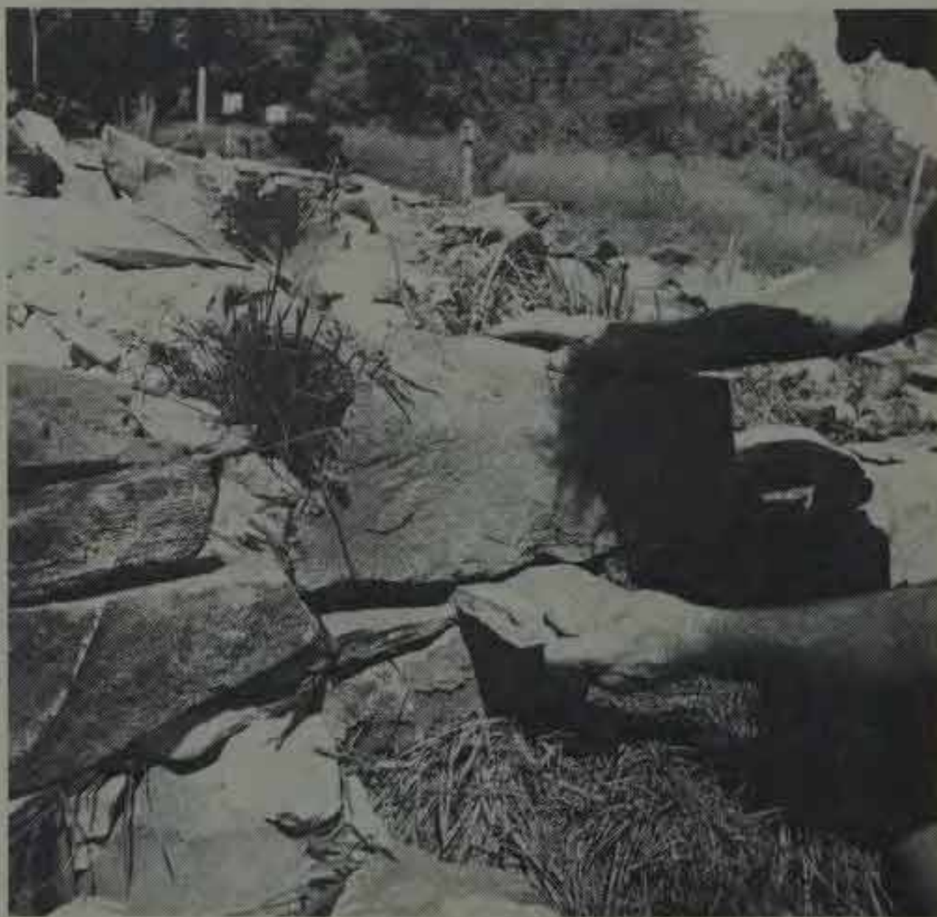
Shimming or chinking the outside of the wall.
