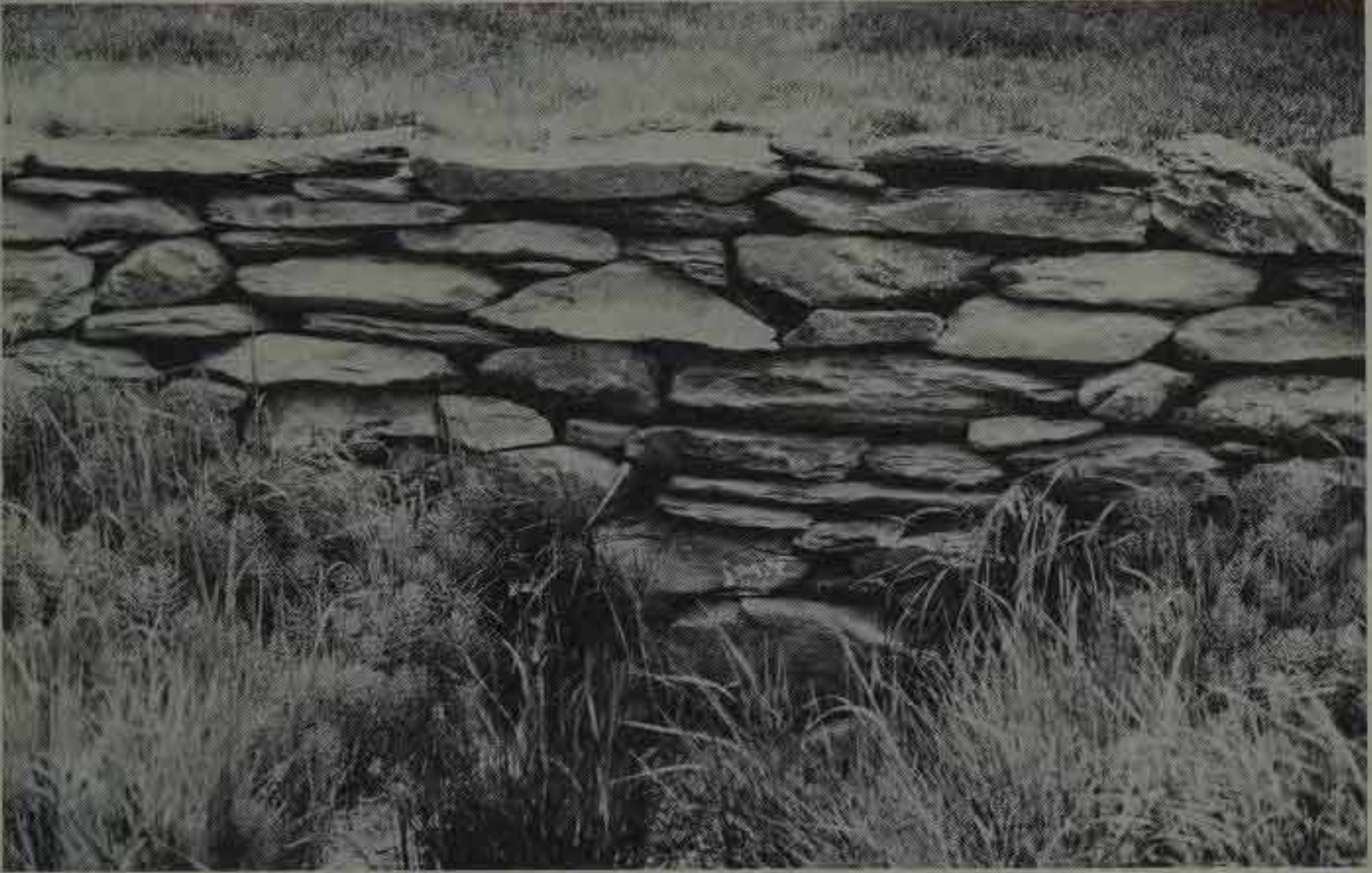
A nicely laid section of wall crosses a ditch evenly.
