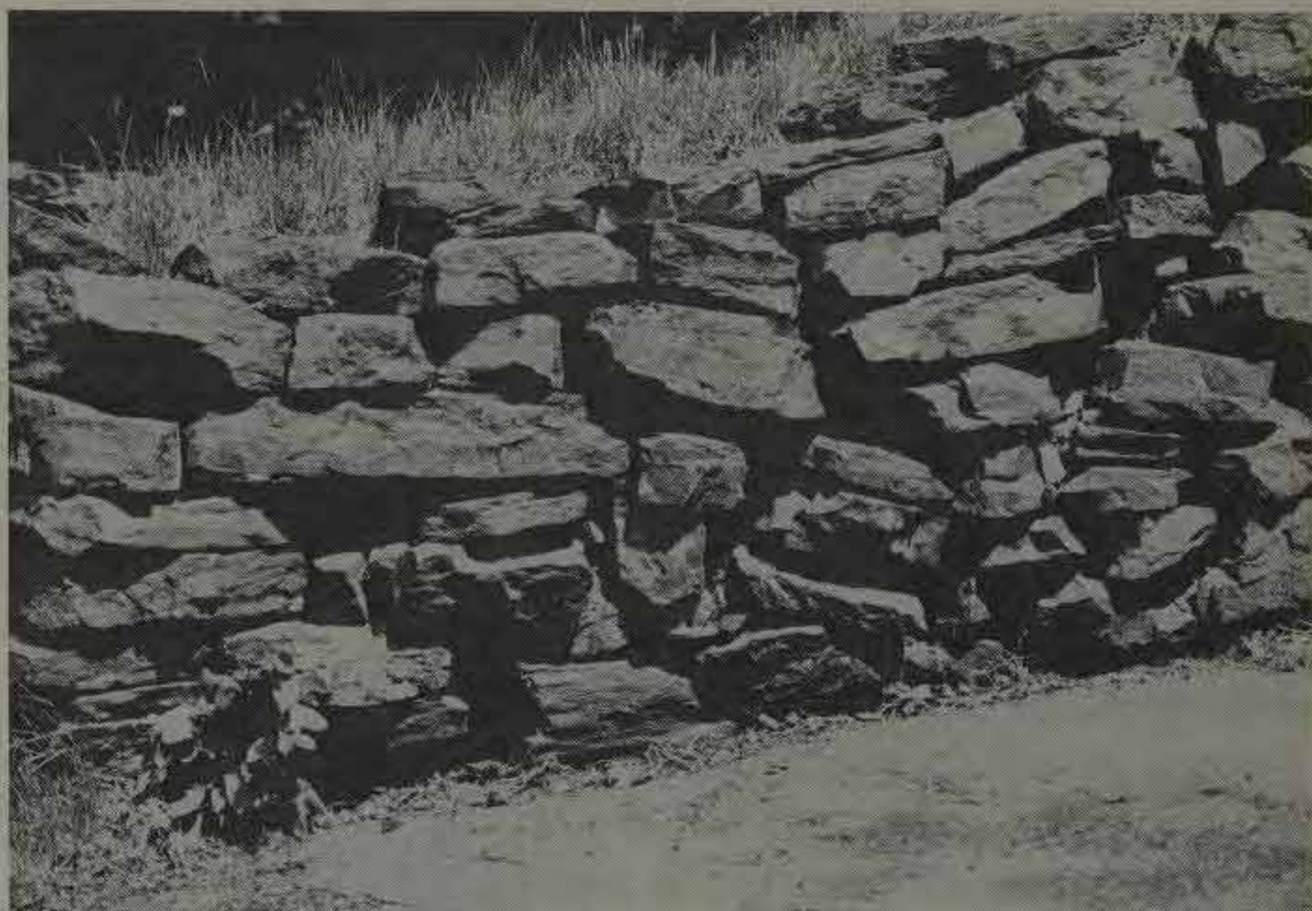
Quarry waste of metamorphic rock provides chunky but good material, in this example poorly laid up.
