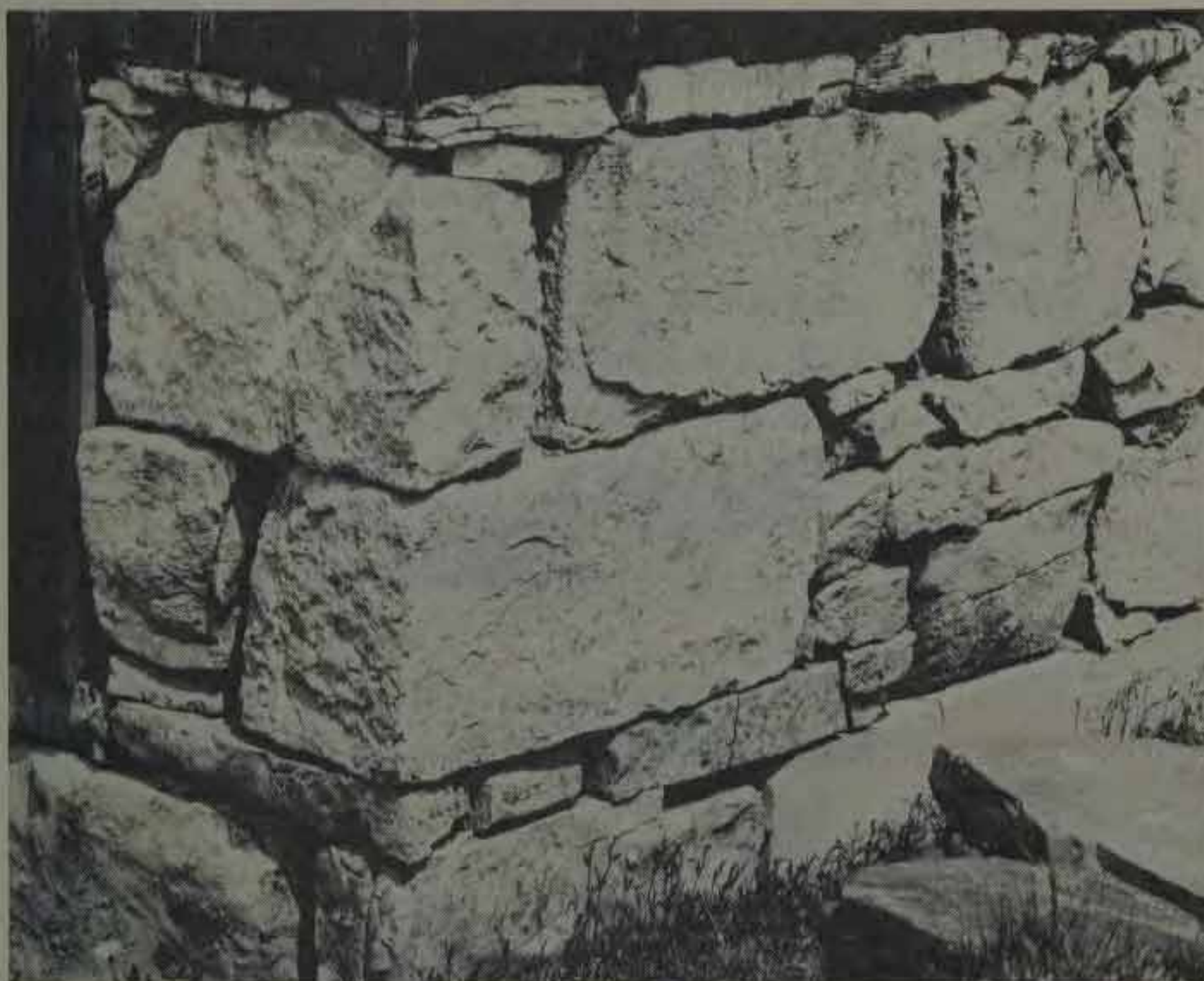
Roughly-dressed stone provides the firm foundation for this old mill.
